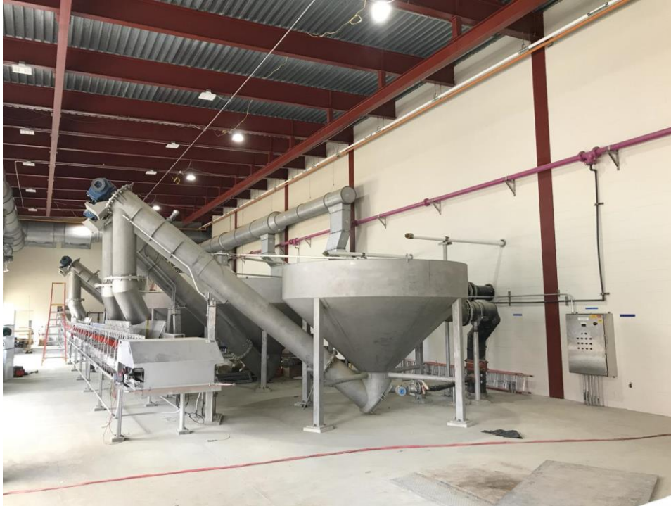
Back River WWTP Headworks Project – GRF Classifiers; September 2020
