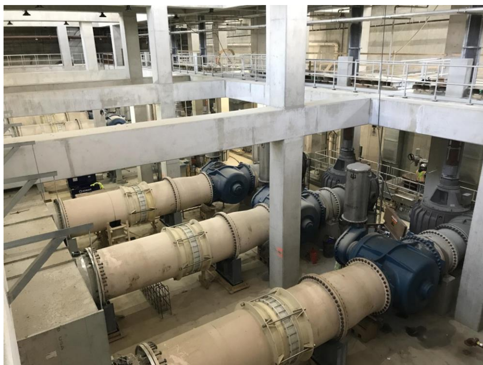
Back River WWTP Headworks Project – IPS Pumps; August 2020
