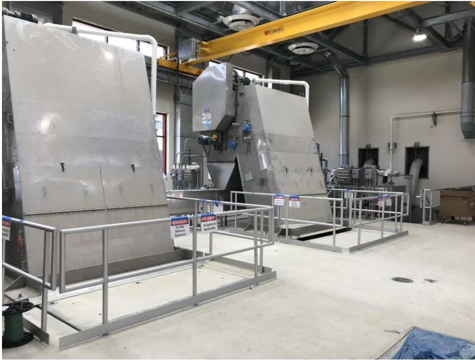
Back River WWTP Headworks Project – Fine Screens Facility; September 2020
